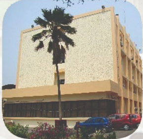
Variable Energy Cyclotron Centre
